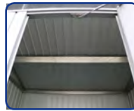
Strong Metal Roof Truss & Structure Carries 20 lbs/sqft Snow Load
