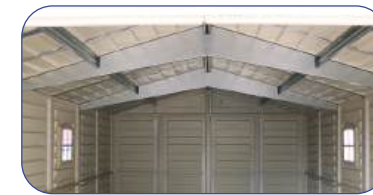
Reinforced steel columns & roof support 120 Kg/ m 2 of snow load
