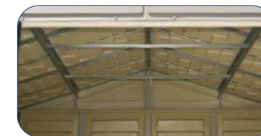
Reinforced steel columns & roof support 100 Kg/ m 2 of snow load
